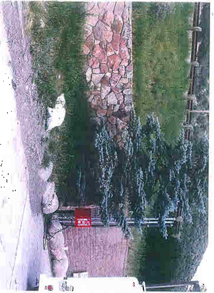
Existing stone veneer and CMU block retaining walls at north edge of site
